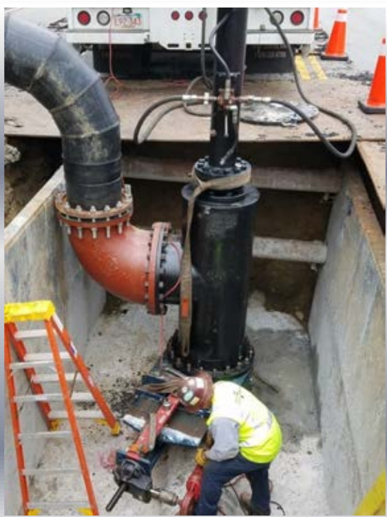
Insertion Valve – South Bedford Street Sewer forcemain Photos by: Brian White, Engineering Division
