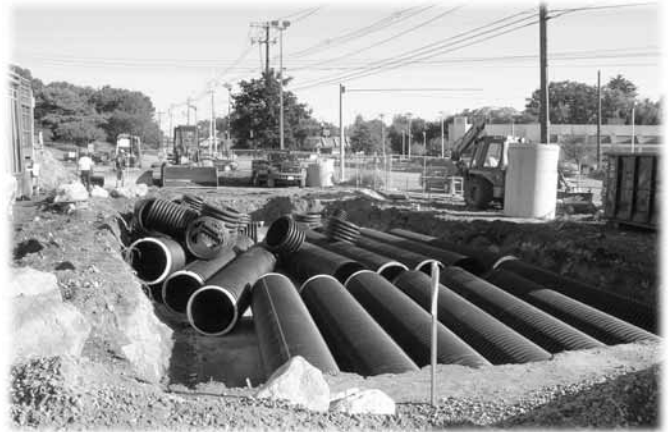
Installing Subsurface Drainage, Burger King Middlesex Turnpike
