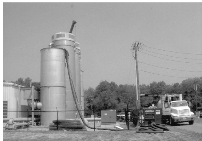
Vinebrook Water Treatment Plant Stripping Towers (Photo by Rosemarie Tieri)
