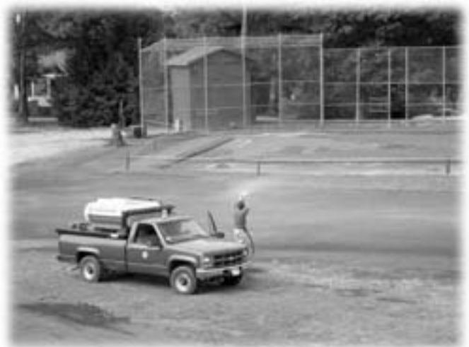
Rich Cote spraying hydro seed on the outfield of the new Little League field constructed at Simonds Park
