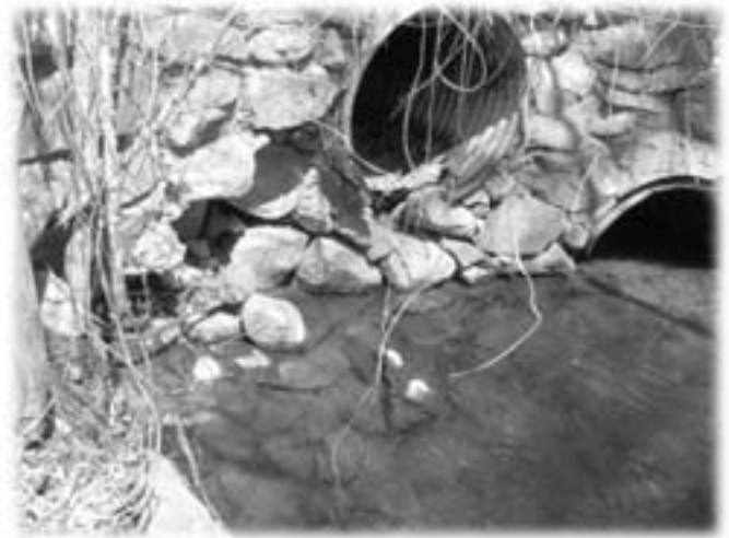
Collapsing stone headwall and corroding pipe
